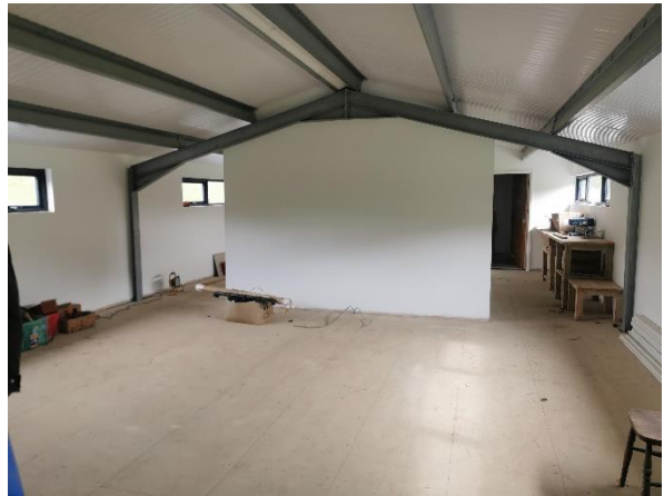
Mezzanine floor space
